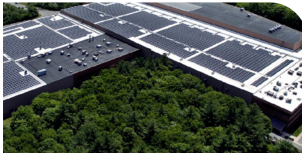
Performance Line Solar Panels Rooftop Installations
